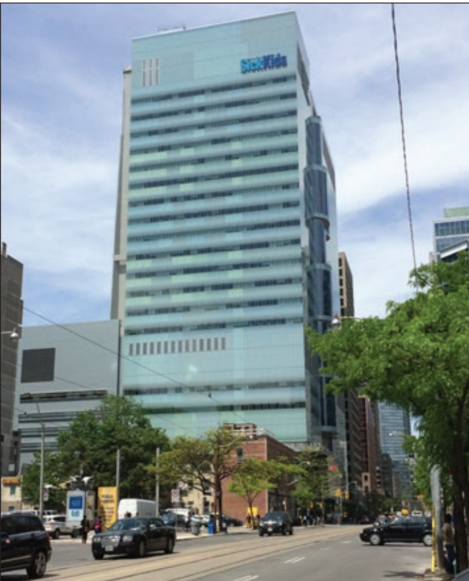
Above, Left: McMaster Children's Hospital in Hamilton, Ontario. More attractive on the inside! Above: Sick Kids Hospital in Downtown Toronto.
